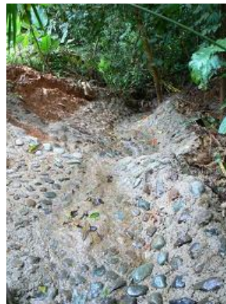
Water drainage head restoration around the Bungalows
