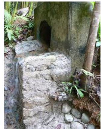
Water drainage head restoration around the Bungalows
